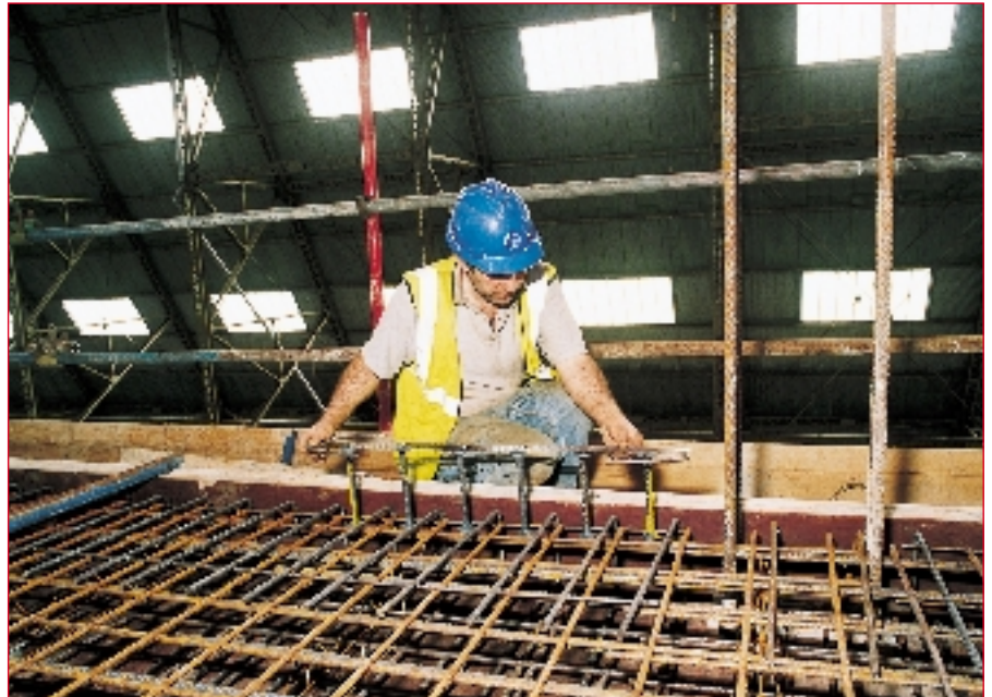
Figure 1: Fixing prefabricated shear reinforcement at Cardington
